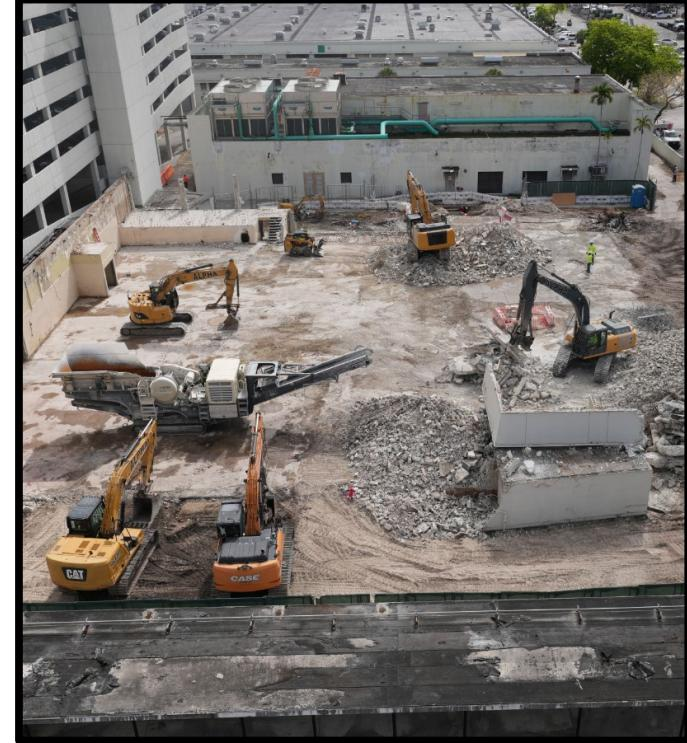
This project involved the demolition of Building No. 3032 including the surrounding concrete canopies and the existing vegetation. Grading and the installation of sod is also included in the work scope. The project will require the removal of significant concrete beams (12"x 30") that extend over a covered walkway and are partially supported by the main columns of Park 2. The demolition began in February 2025 and is targeted for completion by October 2025.
